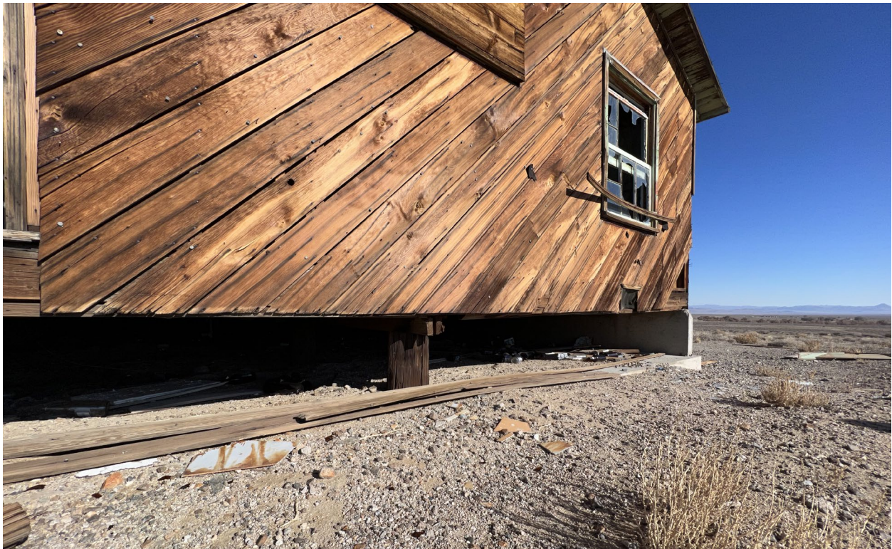
Figure 6. Each Babbitt house sits on a temporary foundation that is open underneath.
